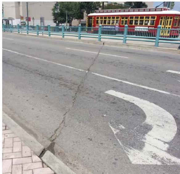
*Above: Cracks in the pavement of lower Canal trace the edges of the fifty-year-old tunnel.*
